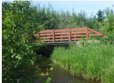
Mill Creek Pedestrian Bridge Replacements
