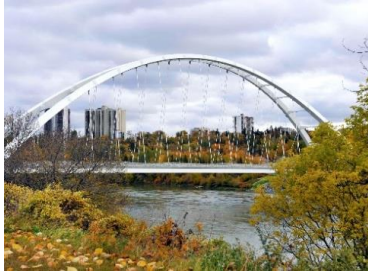
Walterdale Bridge Replacement
