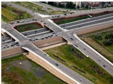
23 Avenue/Gateway Boulevard Interchange
