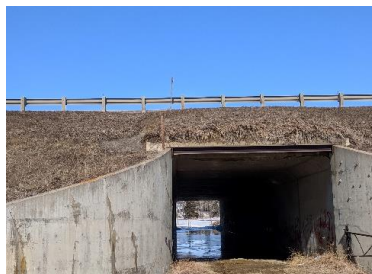
Burman University Underpass
