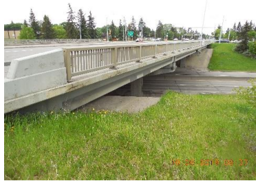
Glenora Overpass Condition Assessment and Rehabilitation Strategy
