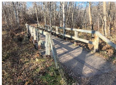
Mill Creek Pedestrian Bridge Replacements
