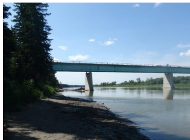
Vinca Bridge Replacement
