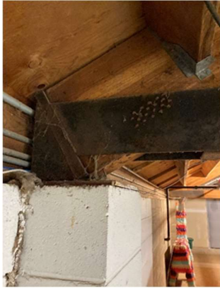
Picture #8.9 – Roof Truss End Joint.
