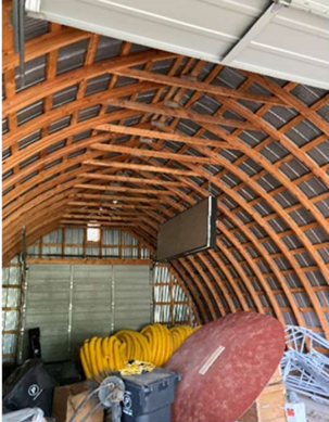
Picture #7.4 – Arch Ribs.
