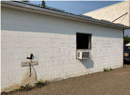
Picture #3.6 – East Wall of Office Side.
