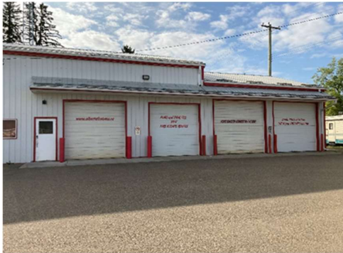
Picture #4.1 – North Side of the Firehall.
