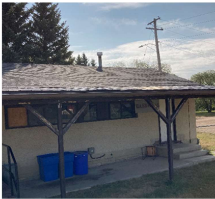
Picture #6.11 - Roof Shingles.
