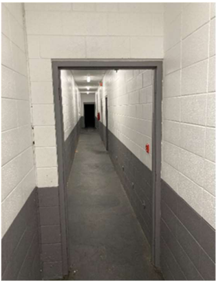
Picture #8.7 – Interior Block Walls of Locker Rooms.
