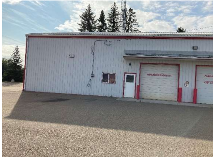
Picture #4.10 – Corrugated Metal Roof.
