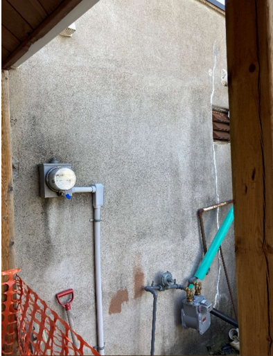
Picture #5.3 – Back Wall Exterior Finish.
