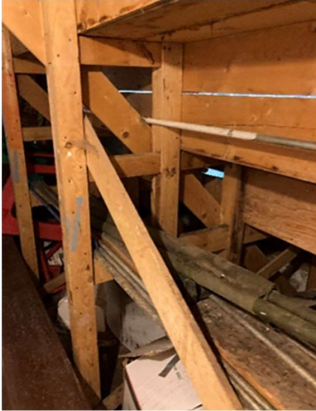
Picture #8.12 – Typical Bleacher Framing.
