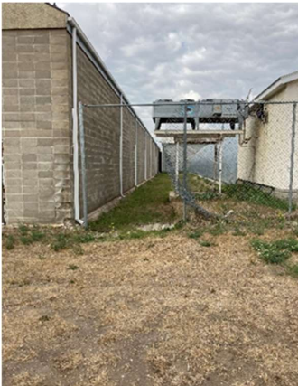
Picture #8.14 – Drainage Ditch Between Arena and the Curling Rink.
