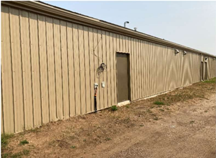
Picture #8.8 – Grading on the South Side of the Locker Rooms.
