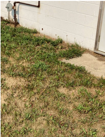
Picture #3.2 - Grading at the Back of the Office.
