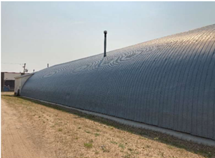
Picture #9.8 – Exterior of Curling Rink Ice Area.
