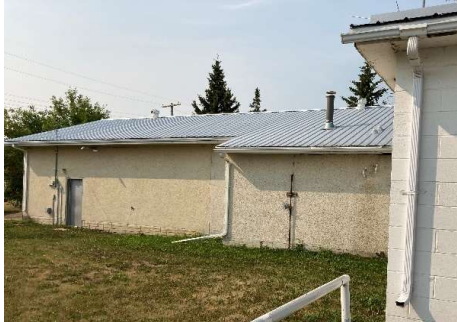
Picture #3.8 – Shop Roof.
