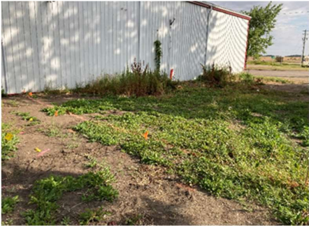
Picture #4.4 – Grading and Landscaping on Southside of the Firehall.
