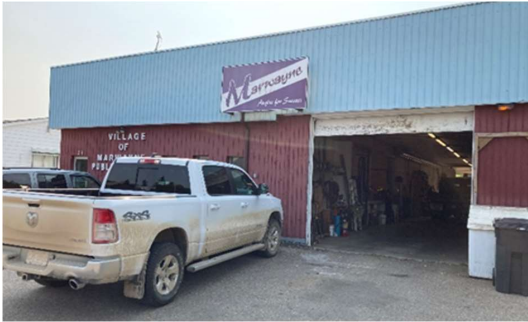
Picture #3.1 - North Exterior Wall of Public Works Office & Shop.
