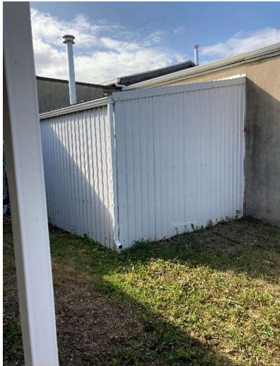
Picture #5.5 – Mechanical Room Lean-to.
