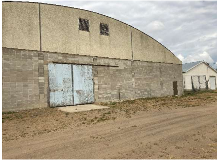
Picture #8.14 – East Wall of the Arena.
