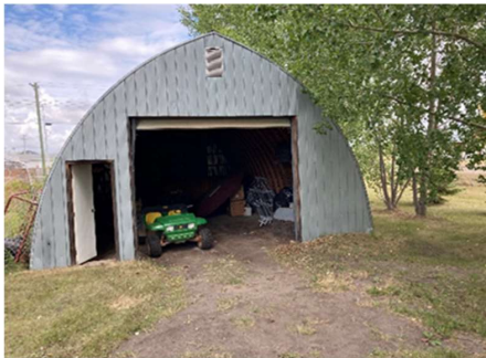
Picture #7.1 – South Side of the Quonset.
