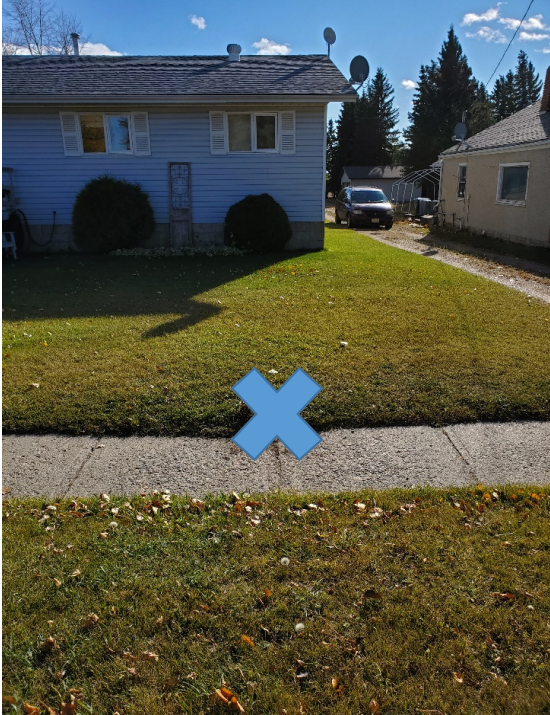
#4. Service line of 23 south 2 nd Street
