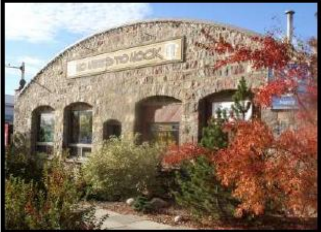
Renovation of Existing Building should be researched and inspected. If material is salvageable, attempts should be made to maintain as much of the original feature as possible
