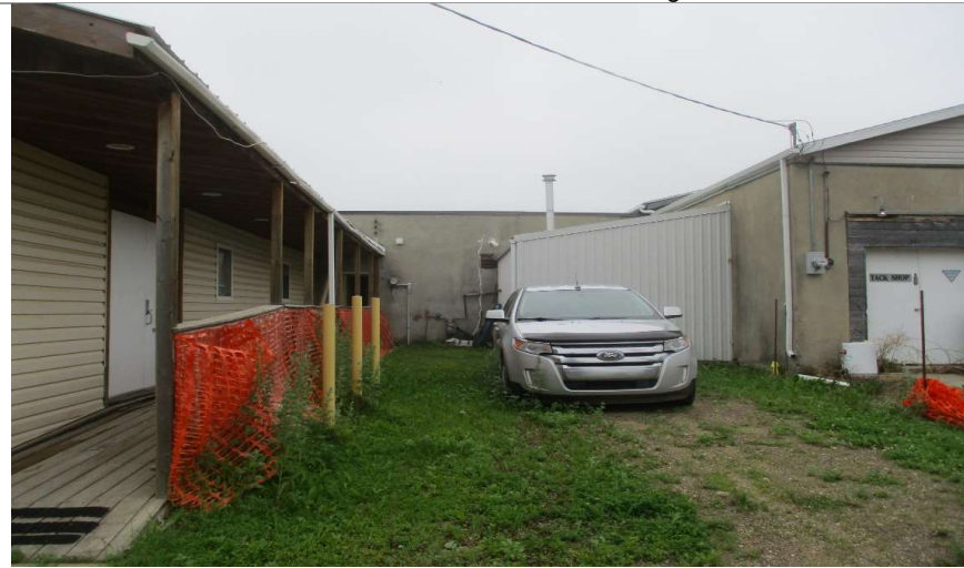
Picture location: Rear of building
