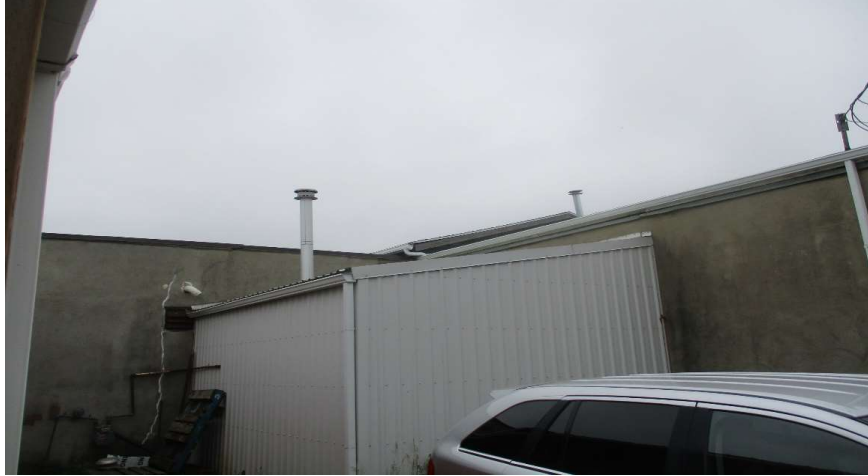
Picture location: Addition
